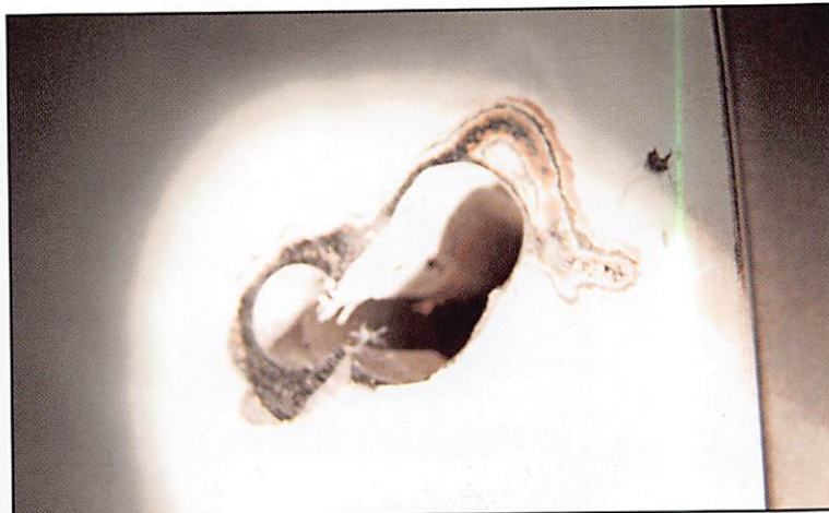
Photo 2, This is the inside of the side wall, although difficult to see the gold colored aluminum barrier layer, it can be seen in the hole.
